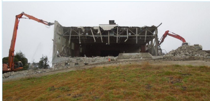
Old Portola Middle School gym being demolished. The new campus will replace Castro Elementary in El Cerrito.
